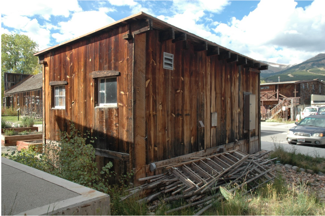
CD 1, Image 78, View to Southeast, of the east-facing and north-facing walls of the shed
