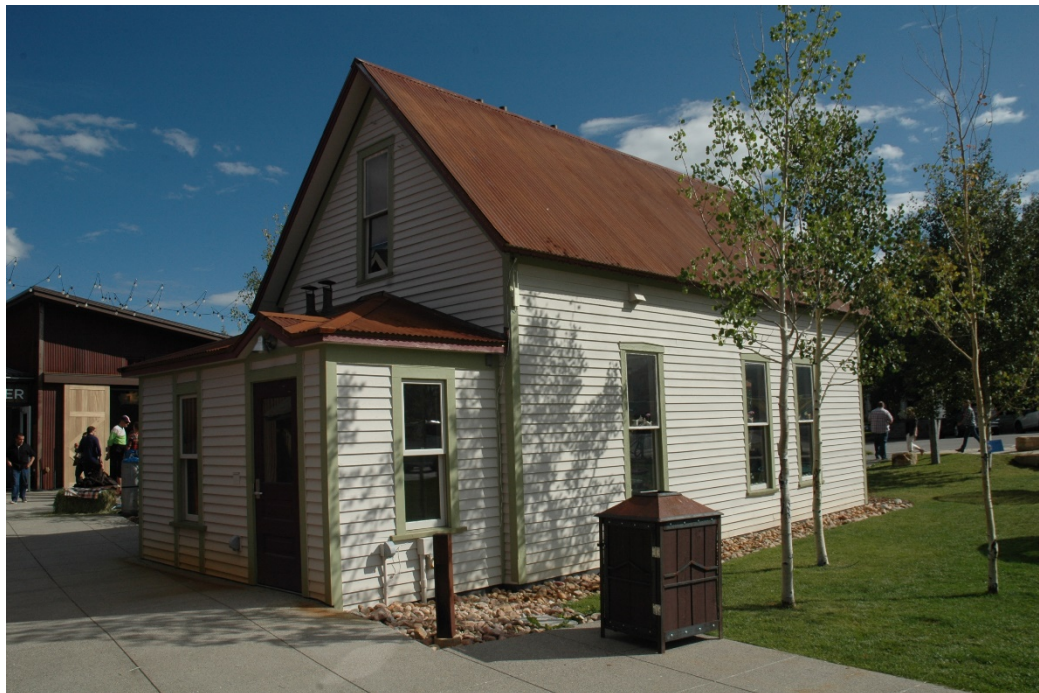
CD 1, Image 76, View to Northeast, of the west-facing and south-facing walls
