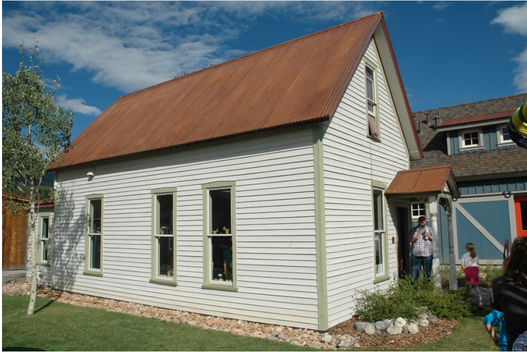
CD 1, Image 75, View to Northwest, of the south-facing and east-facing walls
