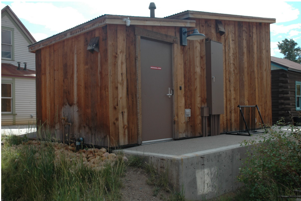
CD 1, Image 77, View to Southwest, of the east-facing and north-facing walls of the Burro Barn / Restrooms building
