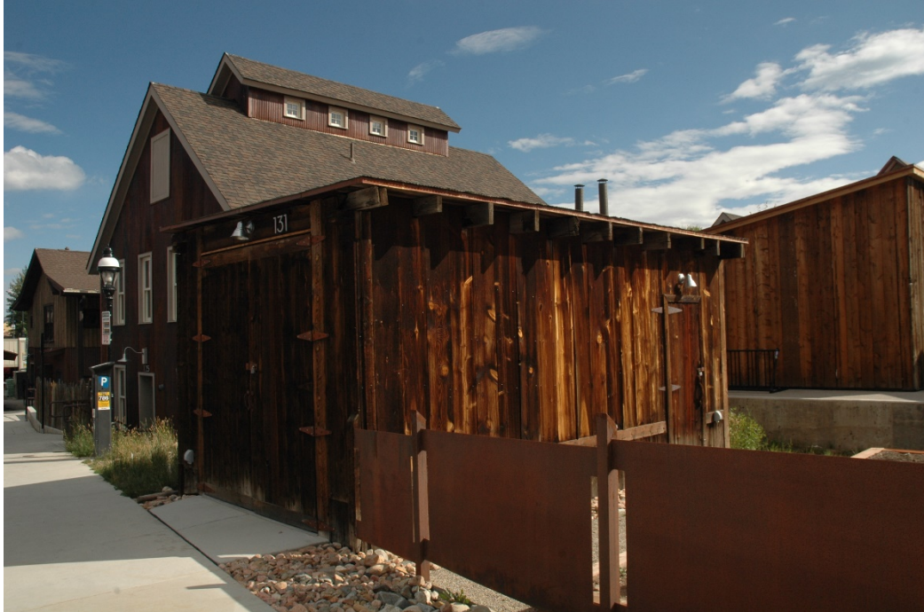
CD 1, Image 79, View to Northeast, of the west-facing and south-facing walls of the shed
