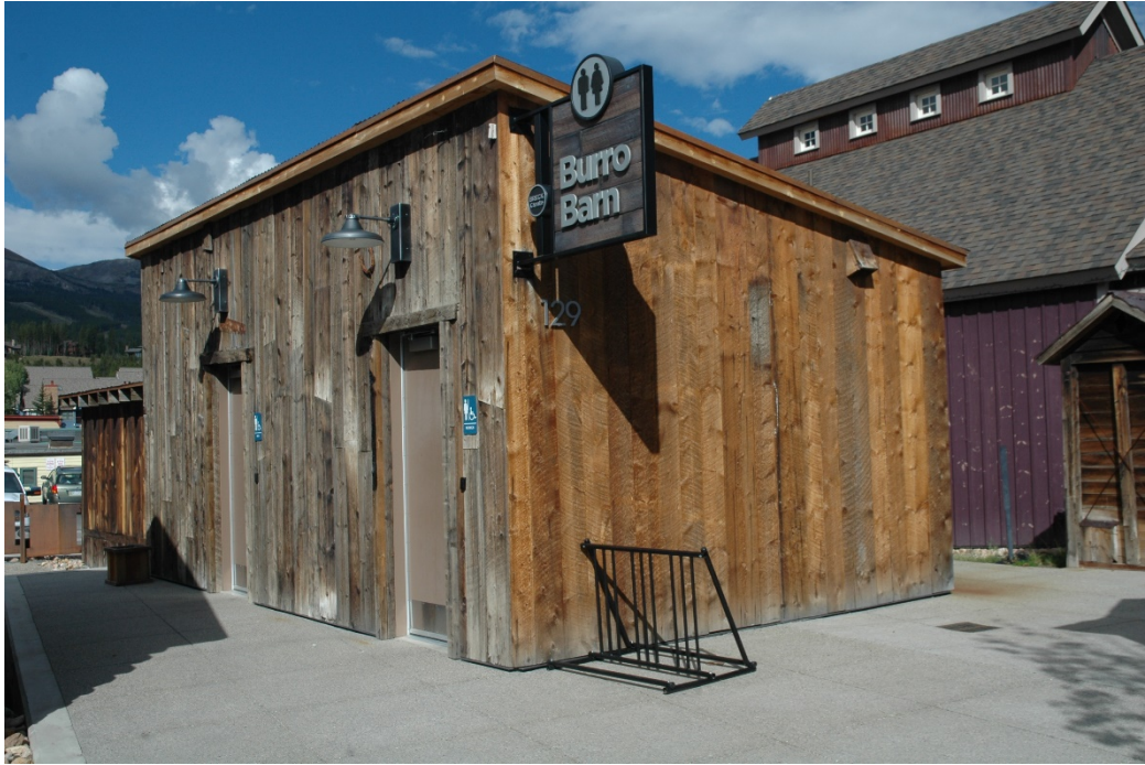
CD 1, Image 73, View to Northwest, of the south-facing and east-facing walls of the Burro Barn / Restrooms building
