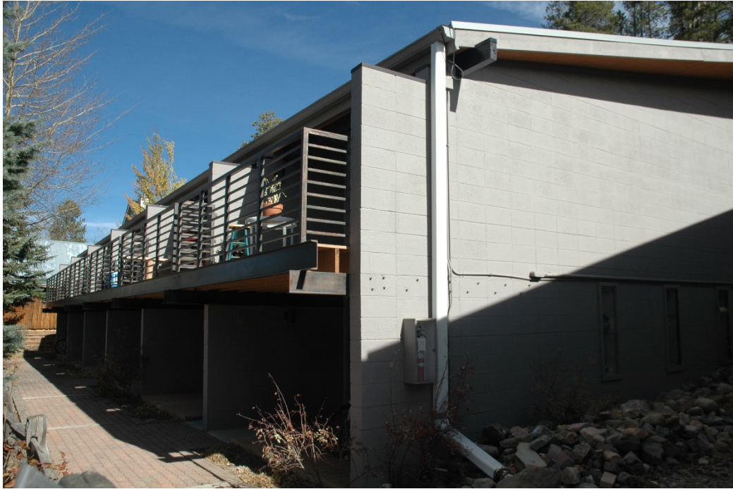
CD 1, Image 28, View to Northeast, of west-facing and south-facing walls of the north building.
