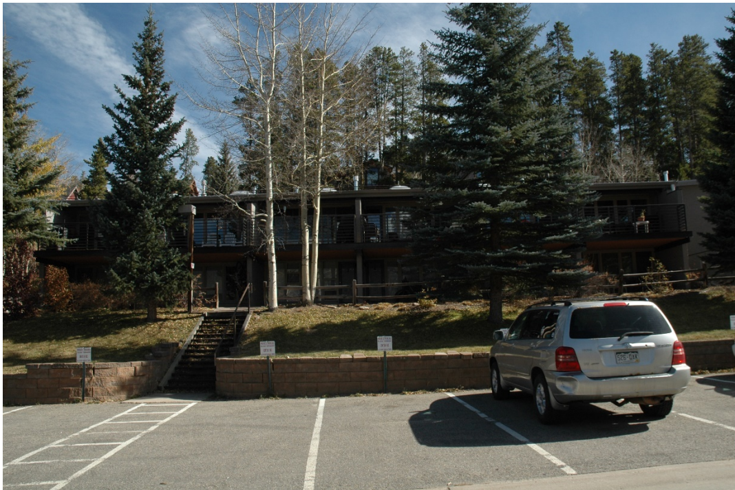
CD 1, Image 27, View to East, of west-facing wall of north building.
