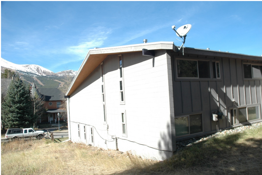
CD 1, Image 35, View to Northwest, of south-facing wall, and south end of the east-facing wall of the south building.
