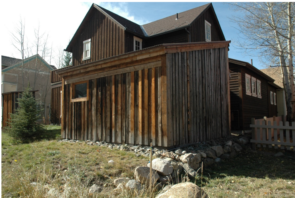
CD 1, Image 16, View to Southwest, of the shed.
