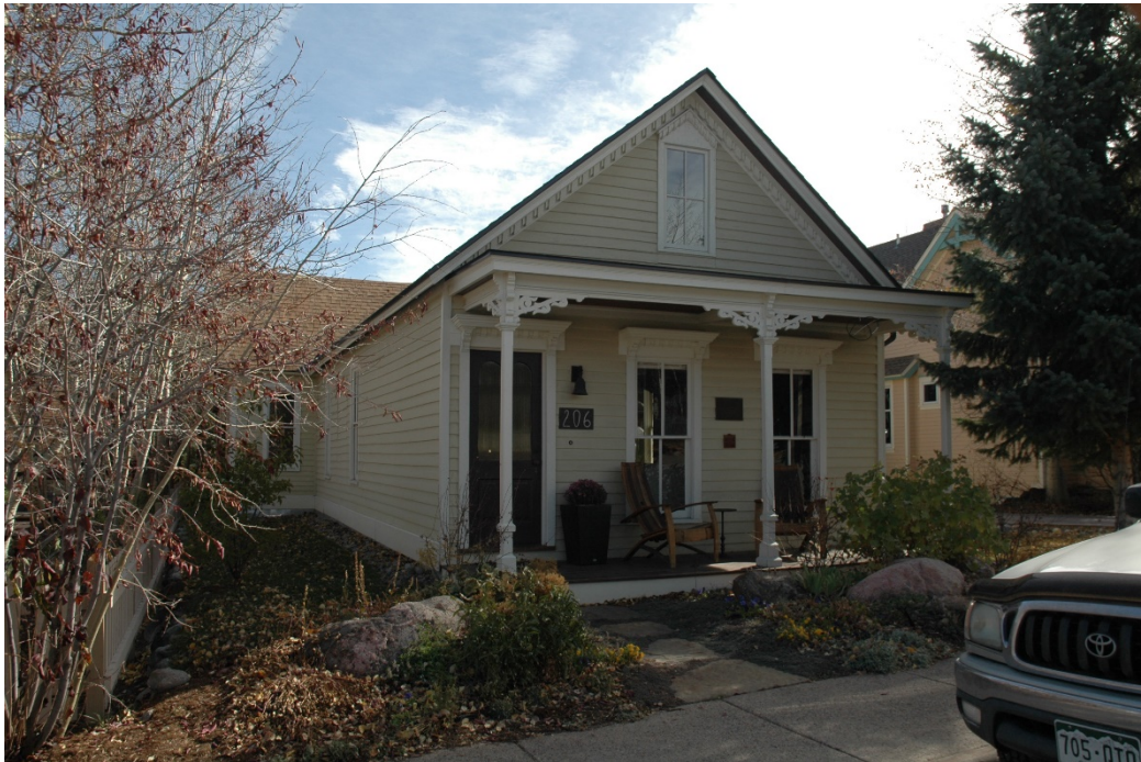
CD 1, Image 9, View to Southeast, of the west-facing (façade) wall and north-facing wall of the original dwelling.
