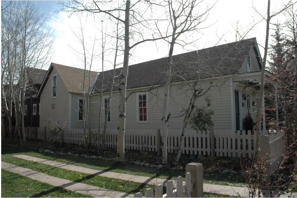
CD 1, Image 10, View to Southeast, primarily of the north-facing wall of the original dwelling.
