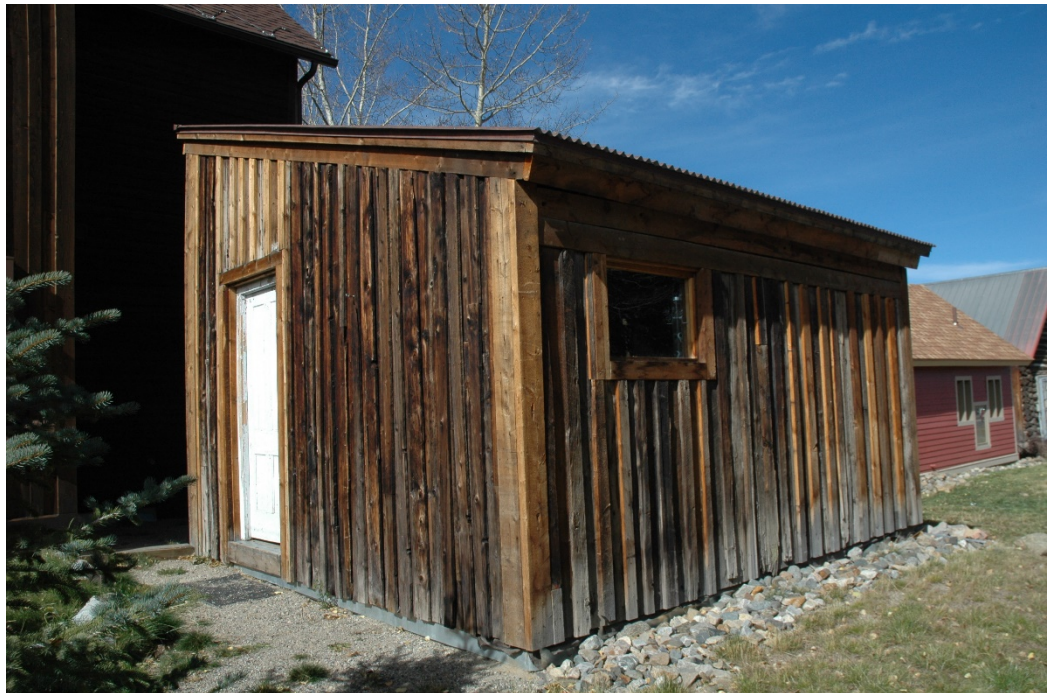
CD 1, Image 15, View to Northwest, of the shed.
