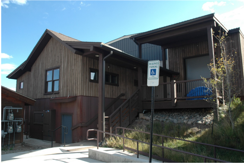
CD 1, Image 61, View to Northeast, of the west-facing wall
