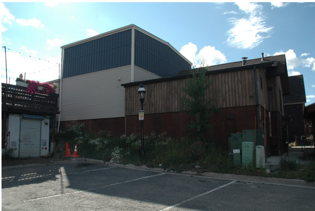
CD 1, Image 62, View to Southeast, of the north-facing wall
