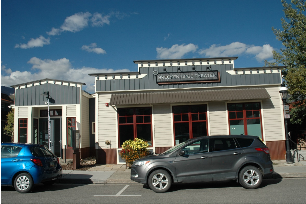
CD 1, Image 57, View to West, of the east-facing (façade) wall
