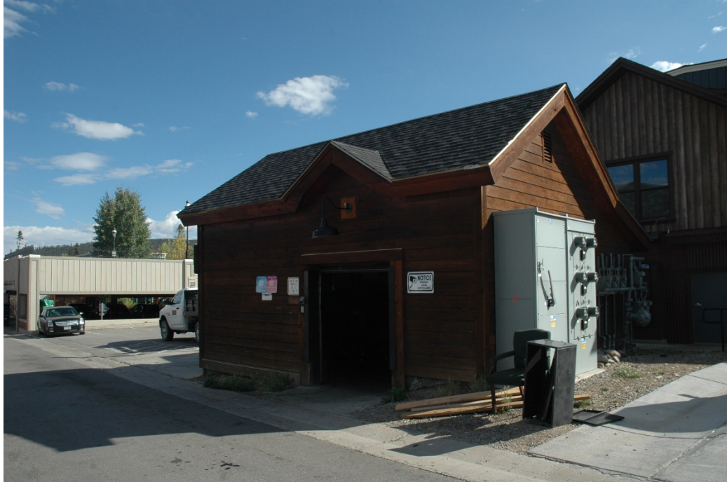
CD 1, Image 64, View to Northeast, of the garage
