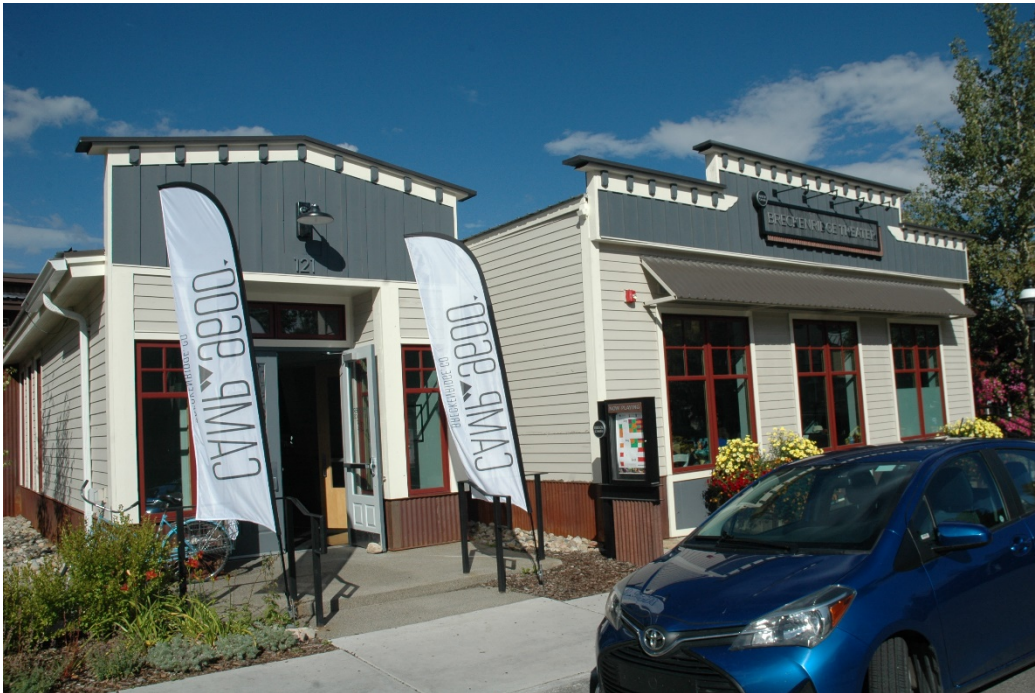
CD 1, Image 58, View to Northwest, primarily of the east-facing (façade) wall
